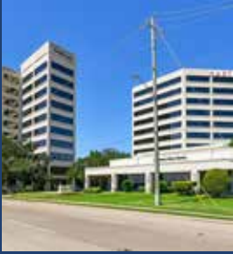
Memorial Tower I & II
